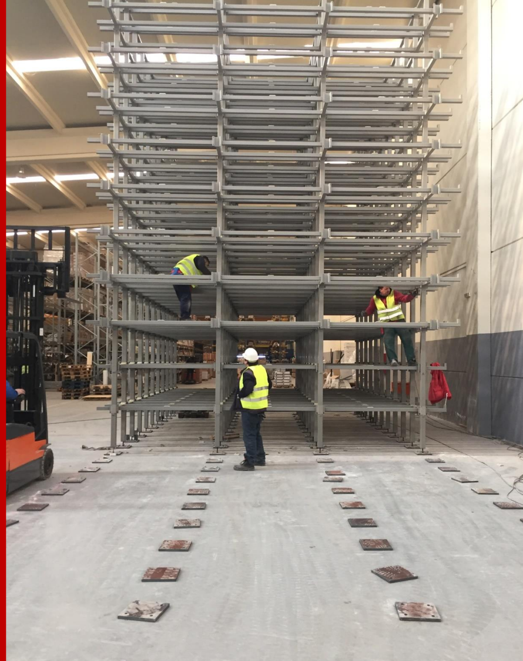
Stacker crane's cells for automated collection of the raw materials.
