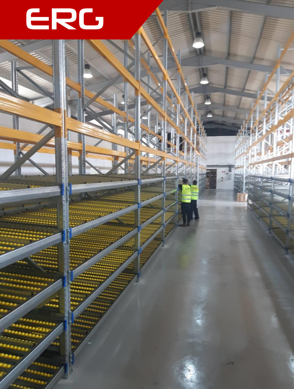
Installation phase of carton live storage.
